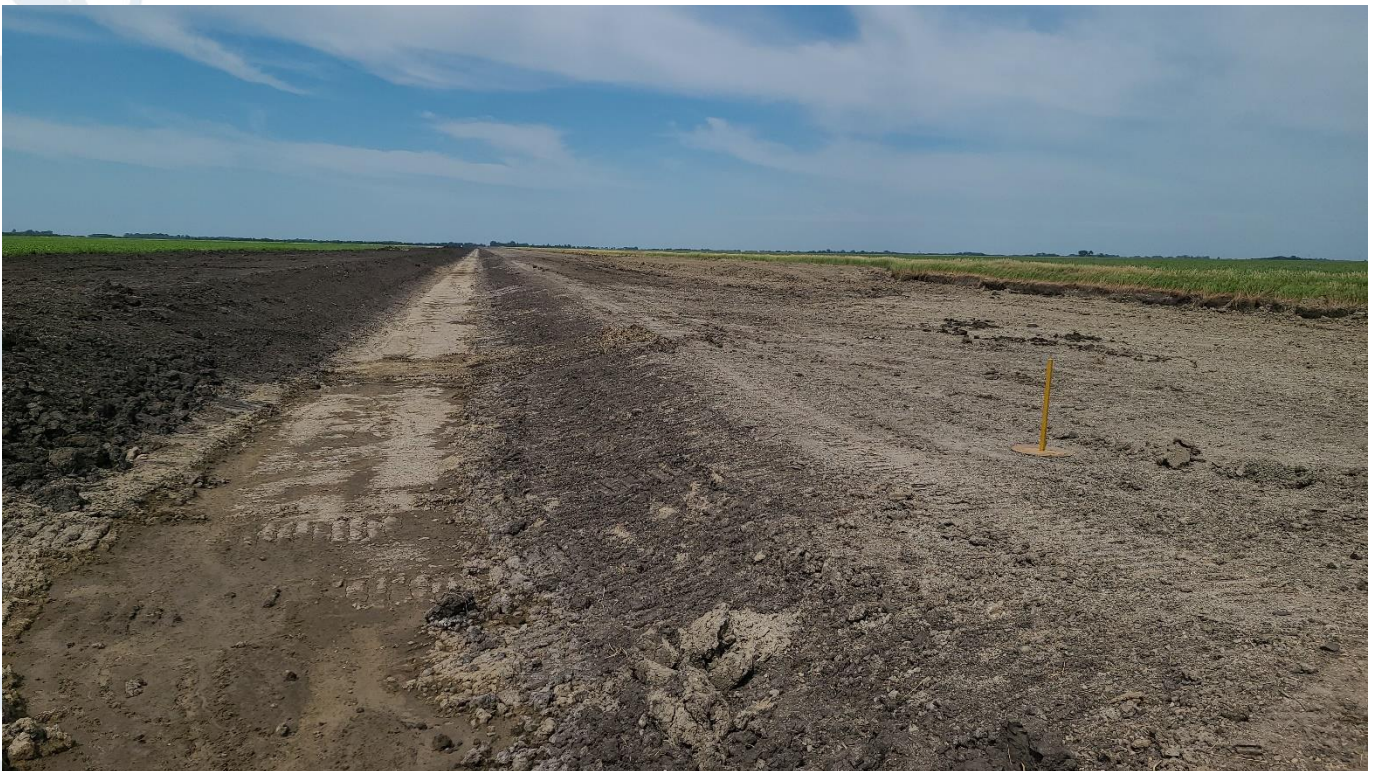
07/14/22: Embankment and Spread Topsoil on Mile 2
