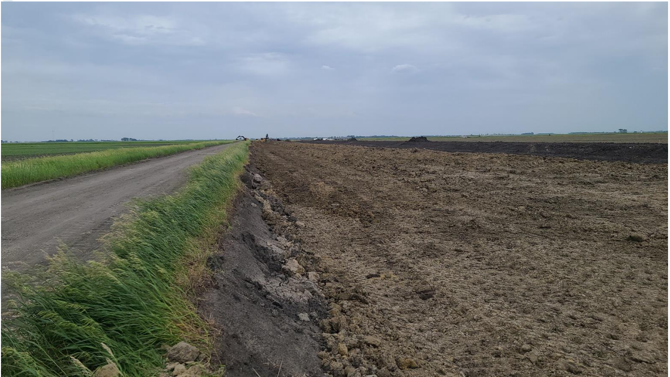
06/20/22: Embankment Placement Along Mile 2.
