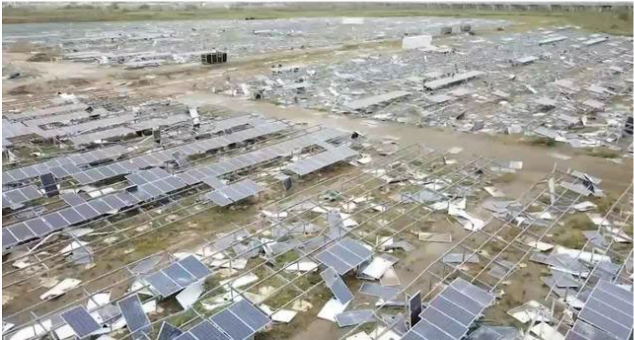
Destroys Solar Farm in Puerto Rico
