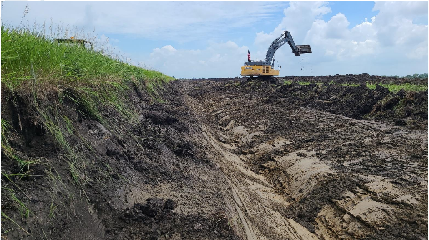
07/07/22: Topsoil Stripping from the Existing Channel along Mile 3
