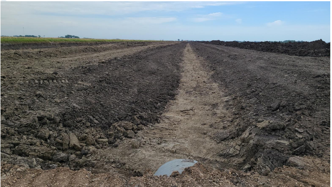
07/14/22: Excavated Channel and Placed Embankment Along Mile 3
