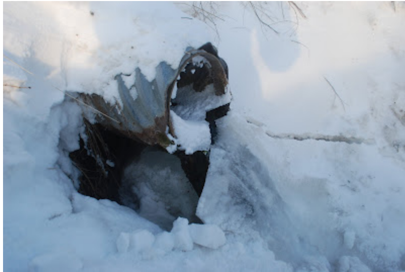
Picture 1. Water continuing to flow out of a tile main on the second-coldest day of 2019.
